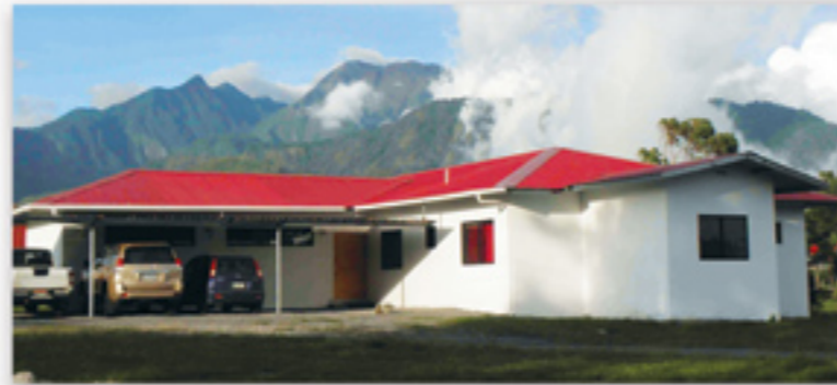
OSOP Headquarters in Panama
